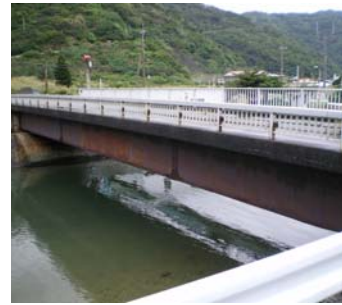
Photo.1 Corrosion Bridge
