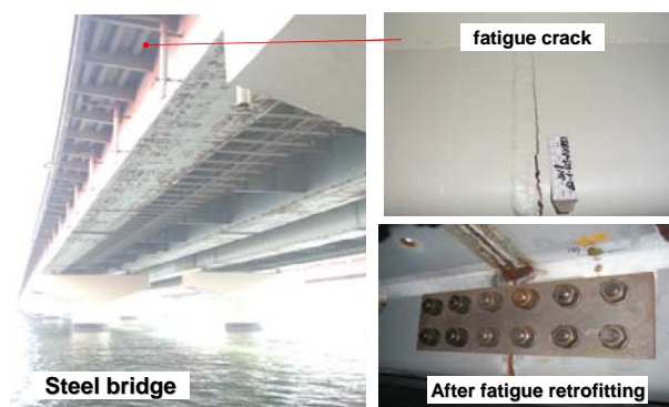
Fig.1 Steel Bridge and Fatigue Retrofitting
